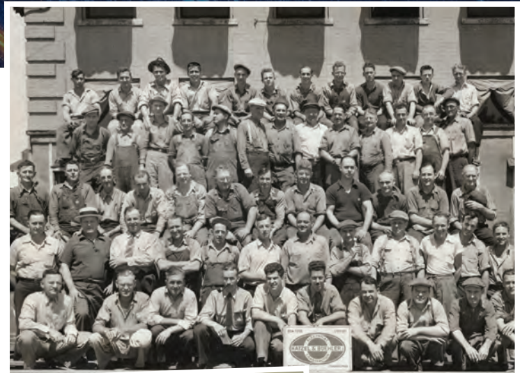
ELECTRICAL WORKERS - TAWA ST. STATION - LANSING, MI - 1939
